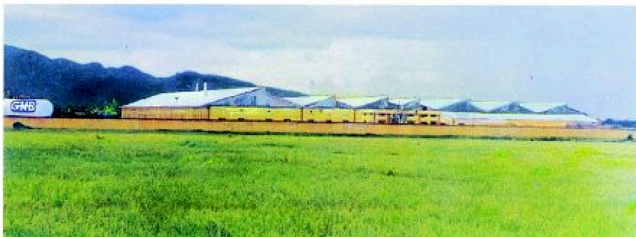
Panoramic view of the GMB factory at Balasore
